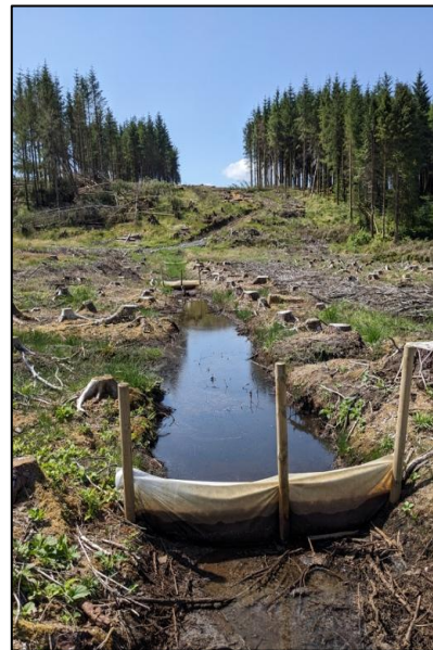
Figure 7: Silt trap for sediment control.
